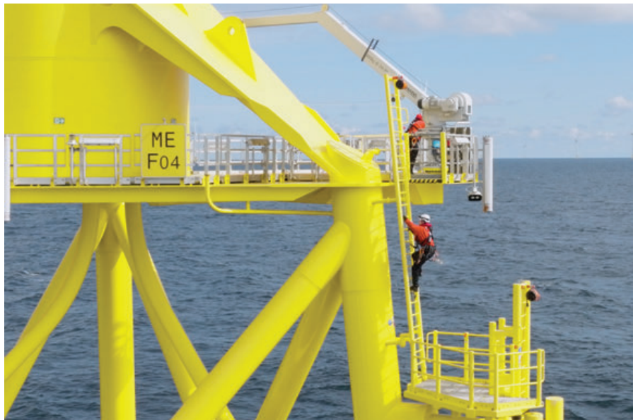
Wind Turbine Technicians at work on Moray East Offshore Wind Farm
