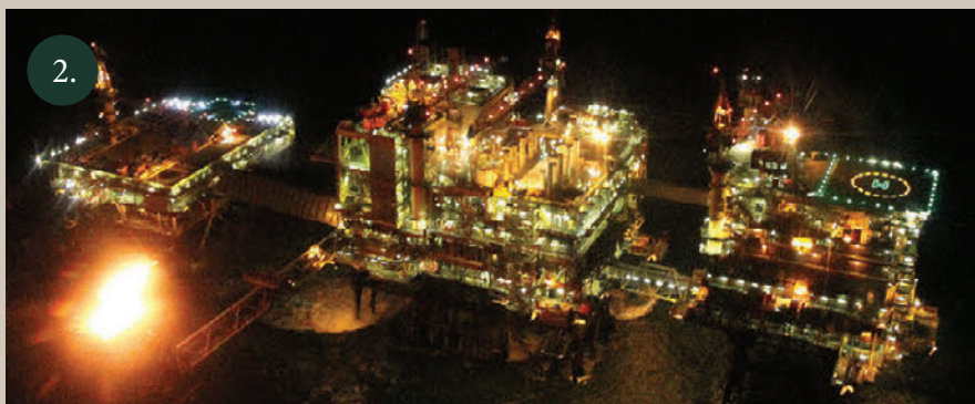
The Centrica CPC1 platform with the new helideck lighting in place
