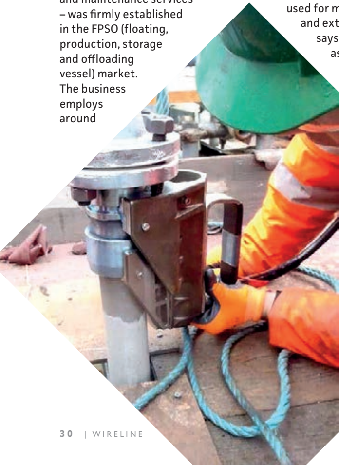
Lokring flanges installed on site
