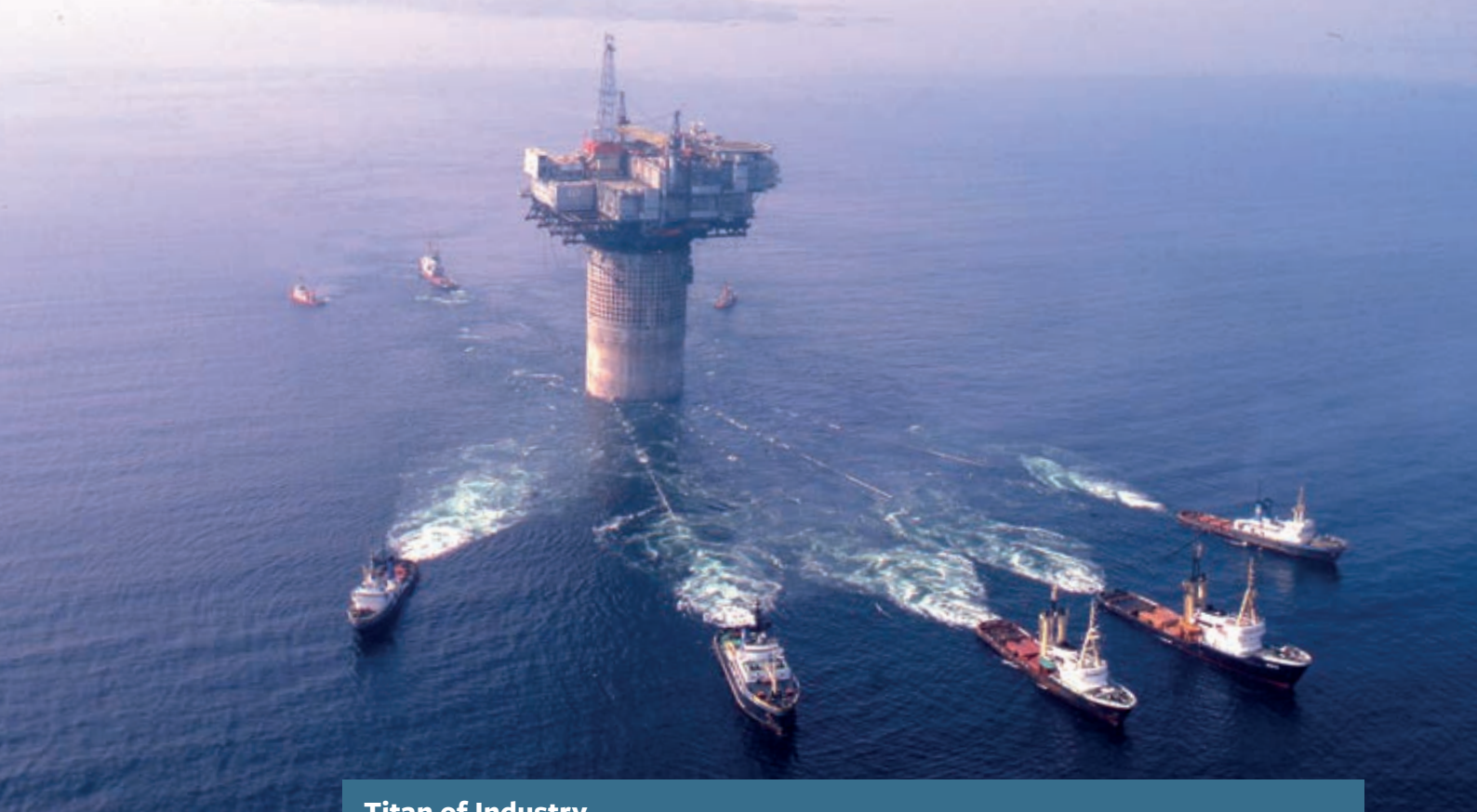
Above: After being built at Kishorn, Yard the Ninian Central platform was towed by seven tugs to its final destination in the northern North Sea.
