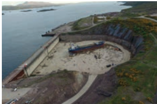
Above: The MV Kaami is towed into the open gates at Kishorn, before water is pumped out to carry out repairs in dry dock.
