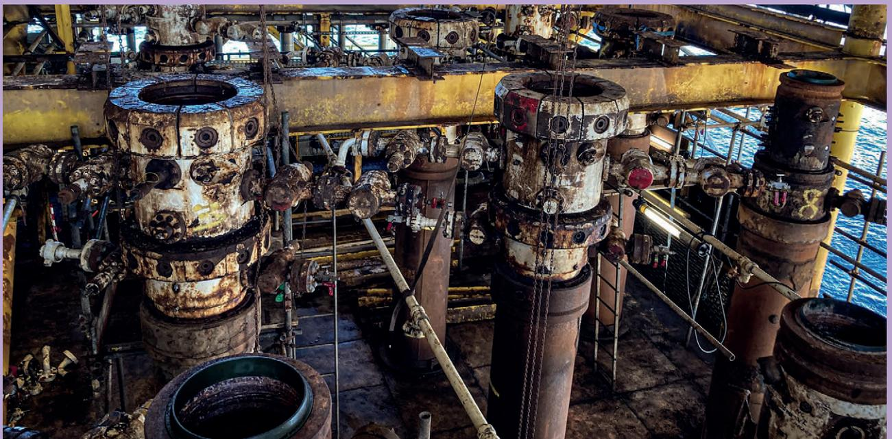
The team took an innovative approach to well abandonment using salt formation as a barrier for zonal isolation. The salt verification process saw the team log 11-3/4in casing with USIT/CBL, before identifying probable halite squeeze locations onto the casing's overall diameter. The salt was then qualified as pressure-sealing, before an internal cement plug was placed.
