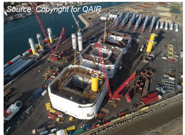
Figure 1: Three floating foundation at Port-La-Nouvelle
