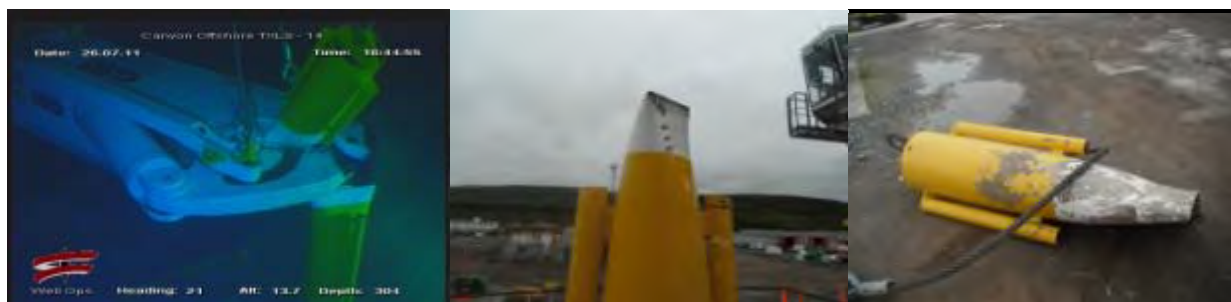
Figure 7-11 Subsea Shearing Operation and final results
