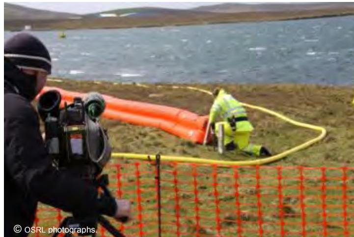
A shoreline boom is erected on shore at Sella Ness while the media watch on.
