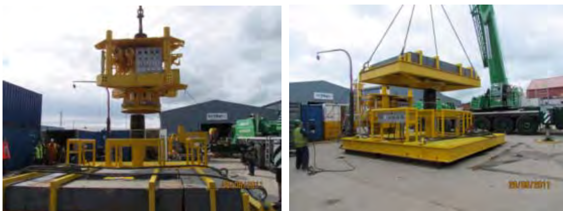
Figure 6-7 Interfacing the pre-loading Structure to the EERD Cap Landing Base
