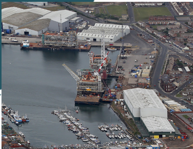
Heerema North Gate Facility
