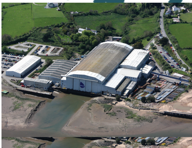
Babcock, Appledore Facility
