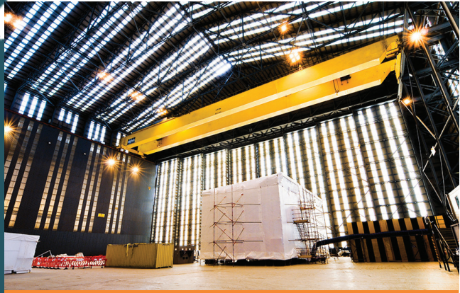
NEP Shop 6 Indoor Fabrication Facility
