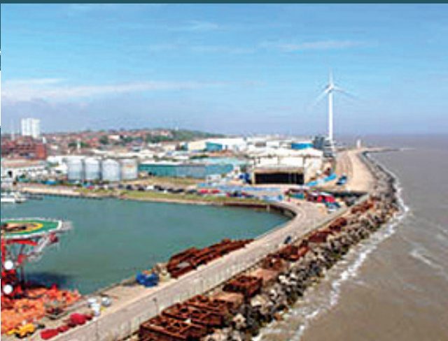
Hamilton Dock North
