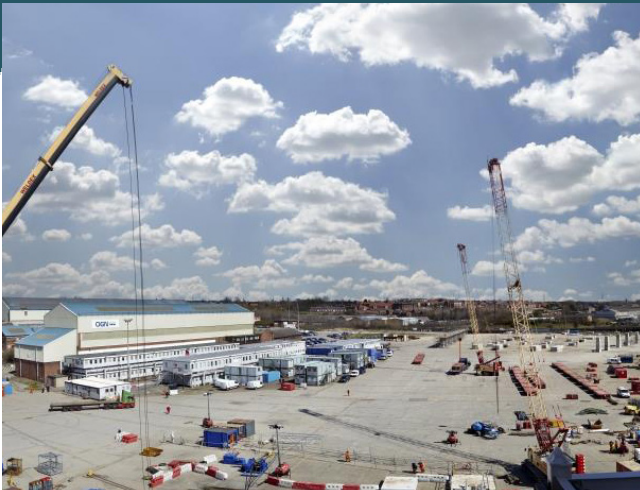
OGN Tyneside Facility
