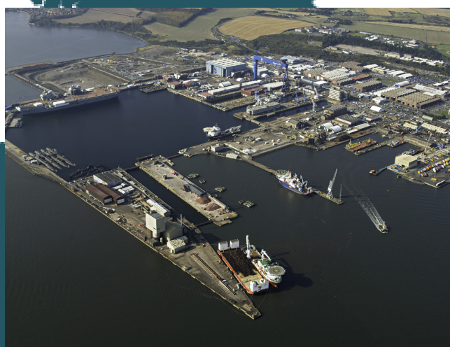
Babcock, Rosyth Facility
