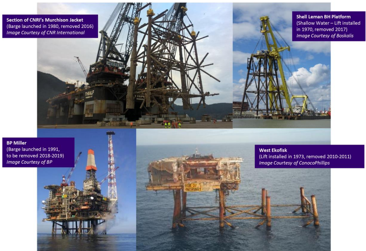
Figure 1 Examples of Steel Piled Jackets in the North Sea Region
