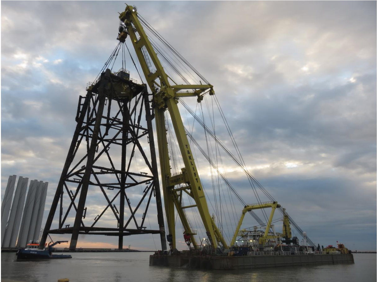
Figure 4: The Lift Vessel Taklift 4 with Shell's Leman Jacket
