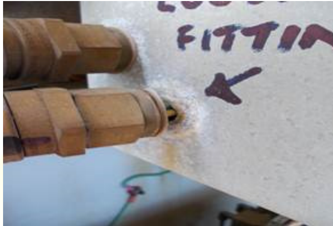
Figure 3 - Example Showing Aluminium Alloy Corrosion which has caused brass adaptor threaded section to break off.
