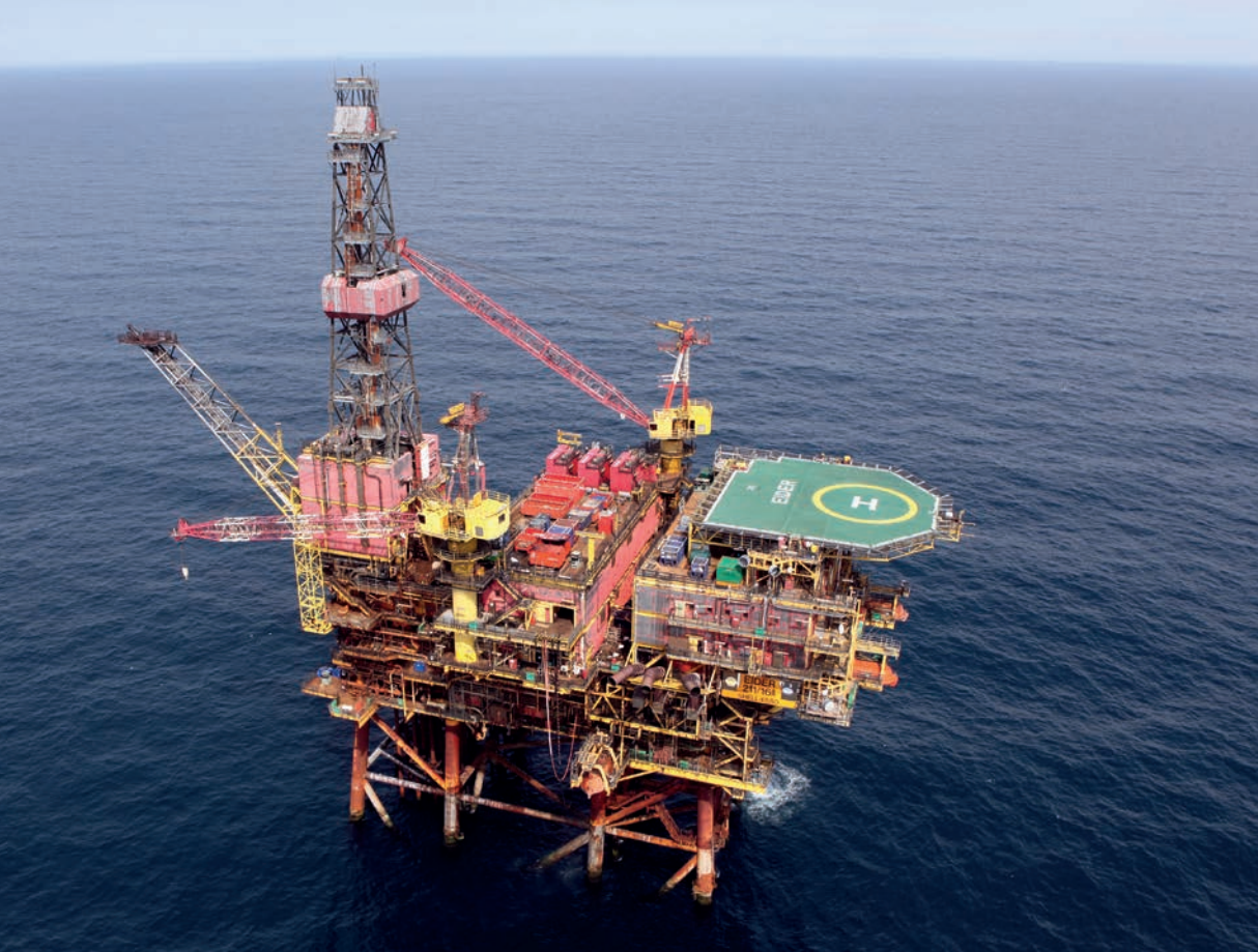
The Eider platform now provides power and system support to the other hub fields.
