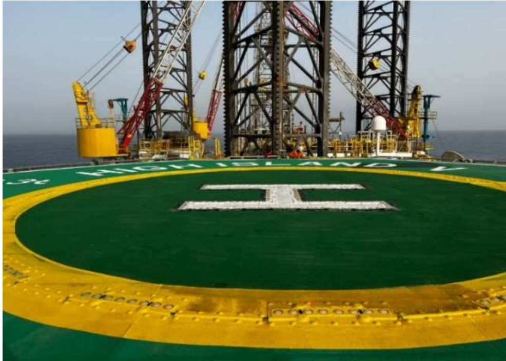
Figure 59: Conventional metal plate deck with friction surface applied.
