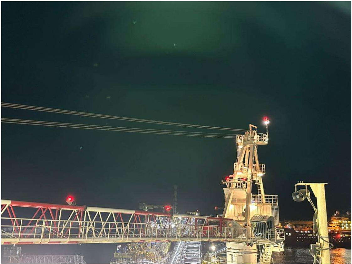
Figure 55: Obstructions lights on a crane and boom
