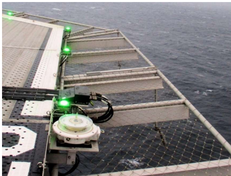
Figure 65: Perimeter net with NDB Long wire Antenna underneath
